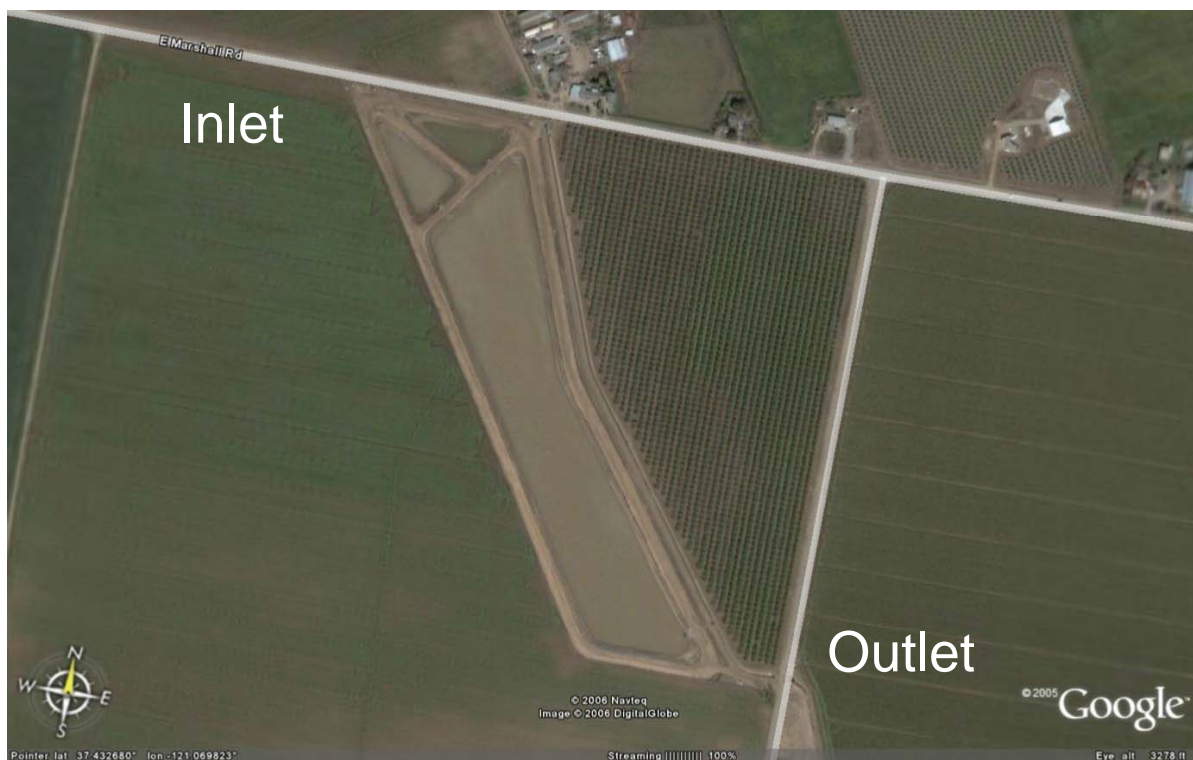
Figure 18: Aerial view of retention pond used for BMP study
